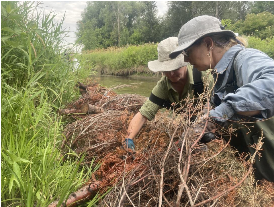
Despite the biting red ants at this site, these volunteers enjoyed completing the eastern wing deflector in Willow Creek.
