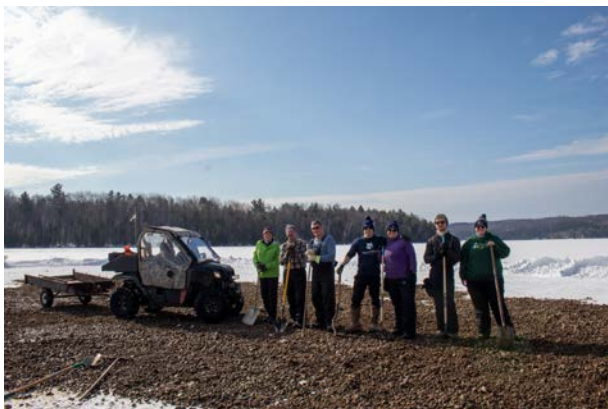
Community members and Watersheds Canada staff work together to spread seventeen tonnes of smaller gravel-sized stone above the historic spawning bed. The stone fell into place with the spring melt.
