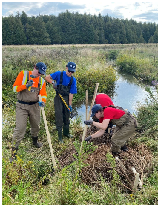
Figure 2. FCC crew build a sediment trap along Squirrel Creek to restore sediment transport balance and improve habitat (September 2025)
