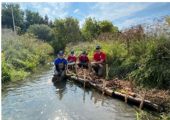
Figure 1. FCC staff with a newly built wing-deflector that will help to restore channel processes at Squirrel Creek (September 2025)
