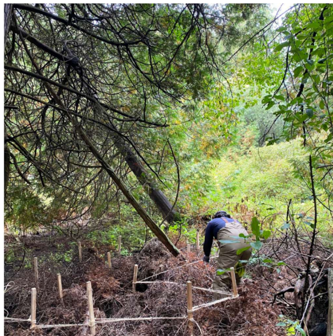
Figure 1. Building a sediment trap in the Marden Creek corridor.
